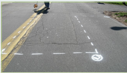
Typical survey paint markings
