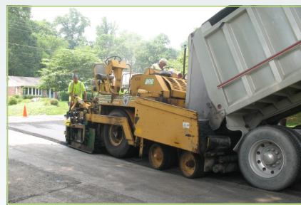
Typical asphalt paving operation
